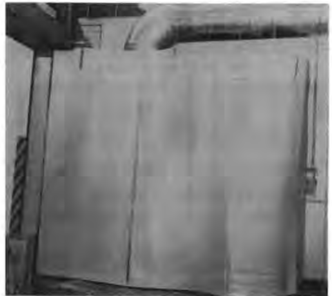
Noise level from machinery is reduced through use of the Eckoustic Noise Barrier.
